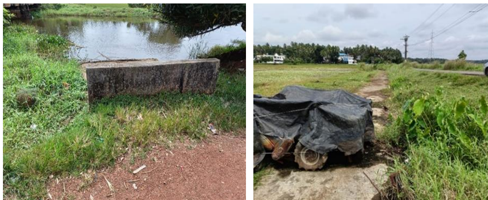
Figure 6: Starting point of concrete slab covering the thodu (a small stream) and the thodu fully covered with concrete slab for the parking area of Killipadam bird watching centre.
