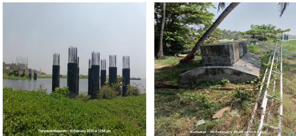
Figure 11: Abandoned Suspension Bridge at Chowara Pozhi.
