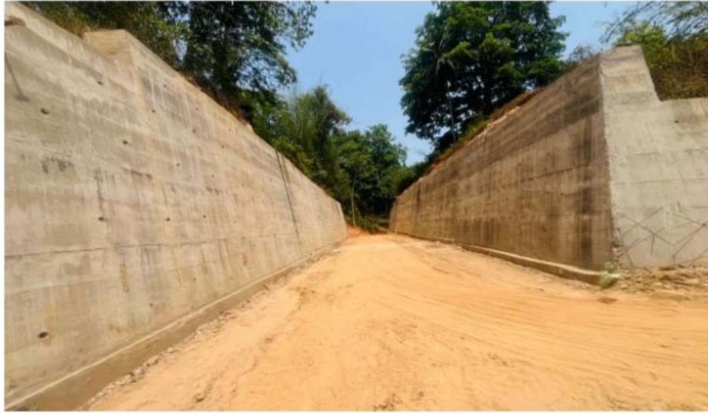
Approach road at Munderi side with breast wall
