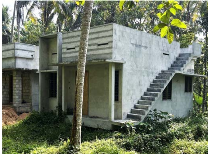
Figure - House construction of TG Beneficiaries in progress (Sreekaryam, Thiruvananthapuram)
