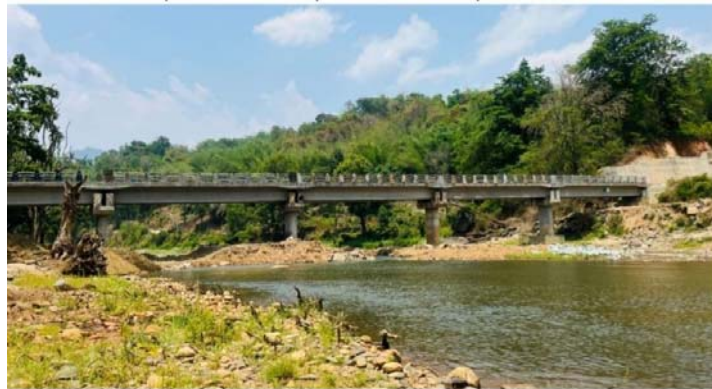
Present stage of bridge
