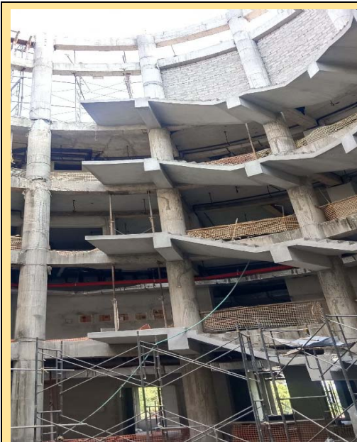
*Inside view of the building
