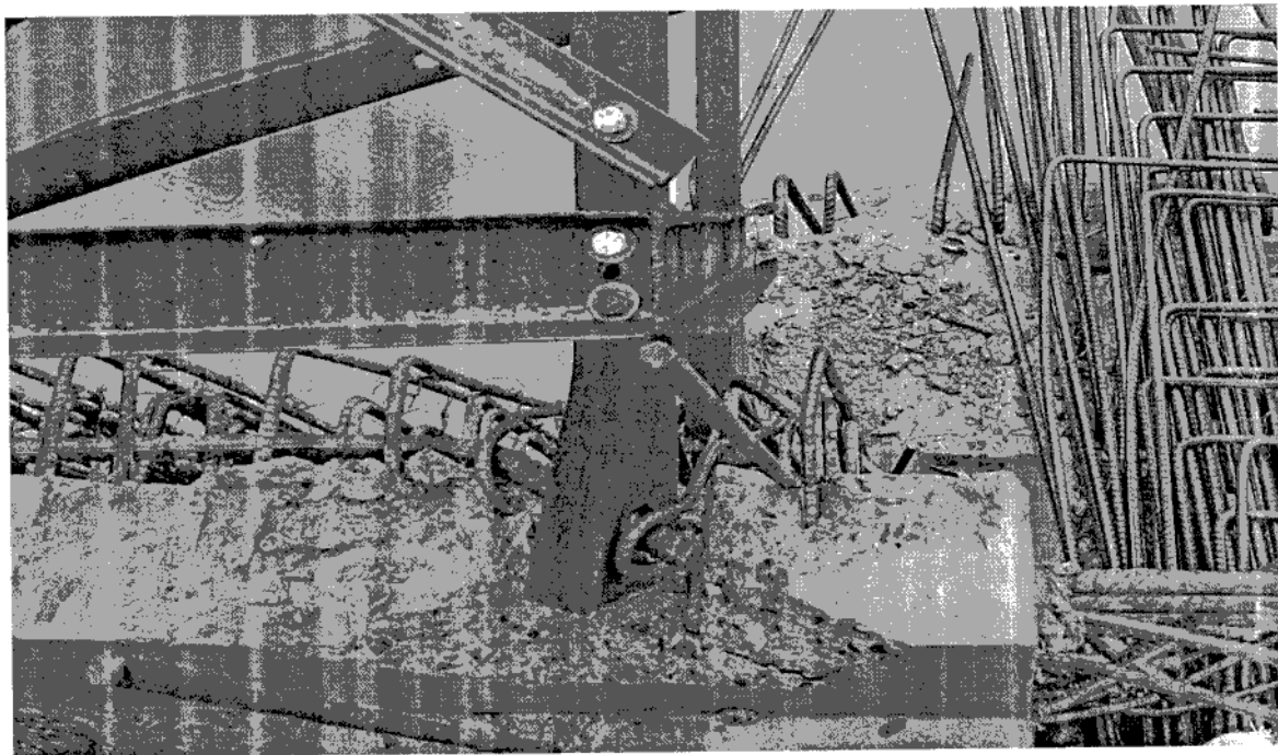
Photo 4 : Cracking and bending of the girders due to fall
