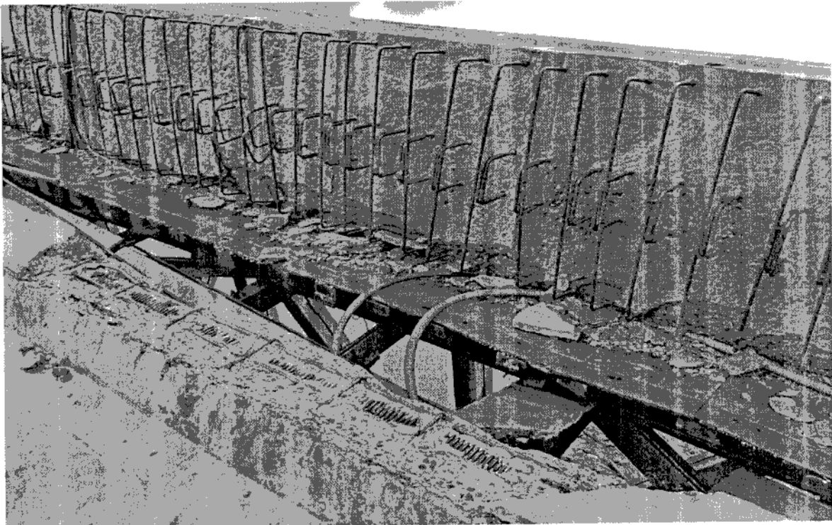
Photo 2: Top view of the girders fallen sideways over the piers
