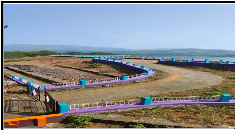
Photo 2.2.2 (ii) : Maintenance and Repainting of parapet wall of Dam
