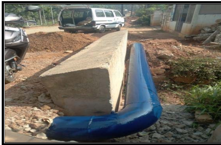
Photo.2.4.3. Replaced GI pipeline
