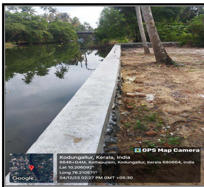
Photo 2.2.5 (iii) : Side protection works to the west bank of Vijayan thodu
