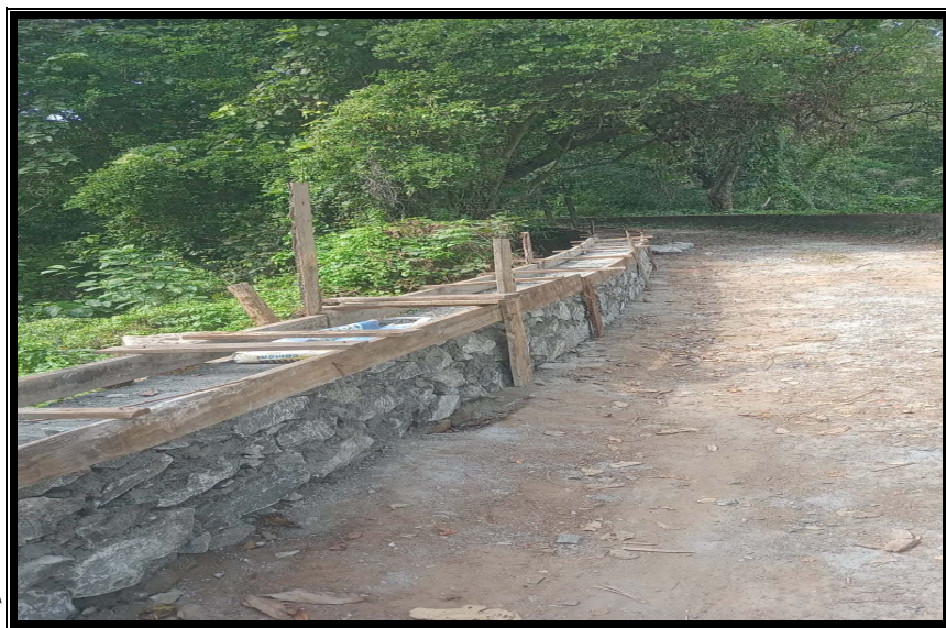
Photo 2.2.3 (i): Rectification of side protection wall
