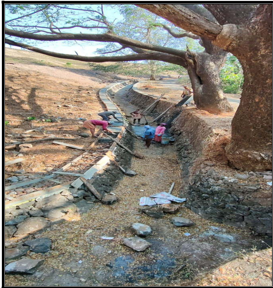
Photo 2.2.2 (i) : Rectification works to the toe drain of Earthen Dam
