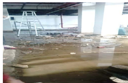
Fig:19 - IIMS - Flooding in the Basement
