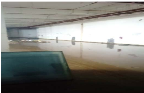
Fig:19 - IIMS - Flooding in the Basement
