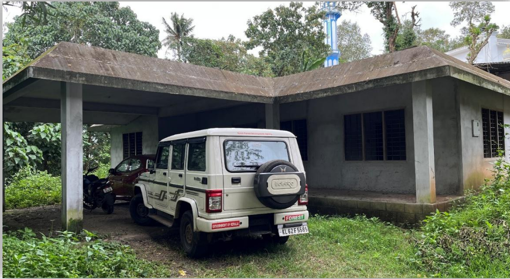
Current state of the construction of Chittar Forest Station building
