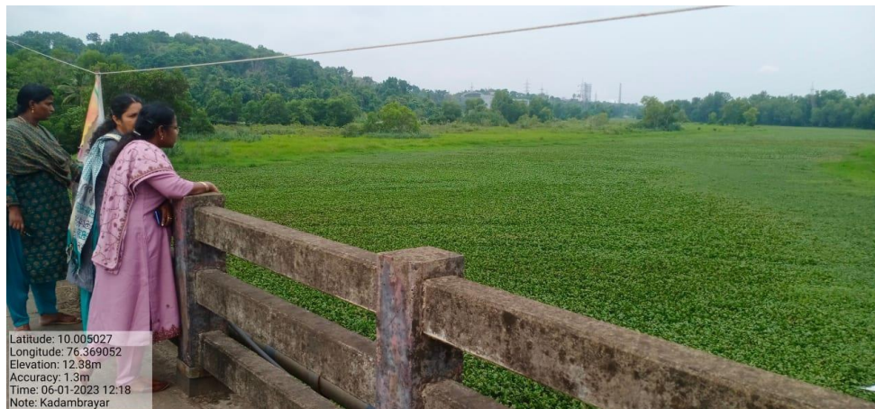
Fig 4 Site visit to Kadambrayar – intake points of four companies in the d/s of the bridge
