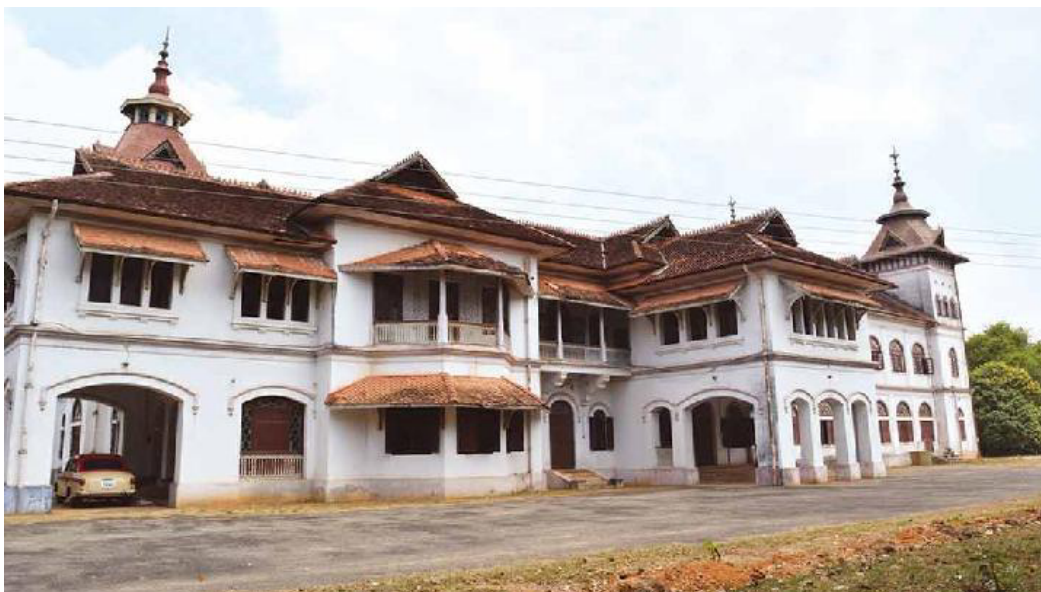
Figure 6.2 The Kowdiar Palace building
