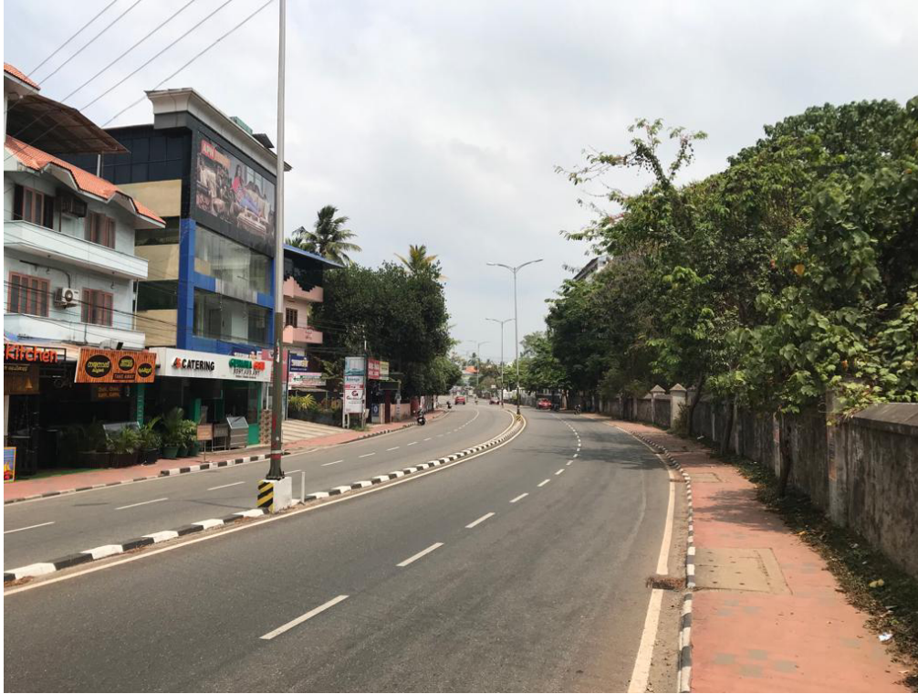
Figure 7.2 : Kowdiar - Ambalamukku Road - potential threat - lacking guidelines to ensure the street character and enclosure quality.
